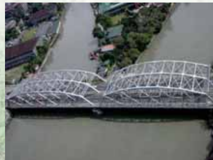
Improvement of Existing Bridges along Pasig River and Marikina River, Philippines
