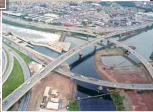
Environmental Improvement Project
