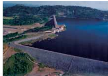
Bili Bili Multipurpose Dam Project, Indonesia
