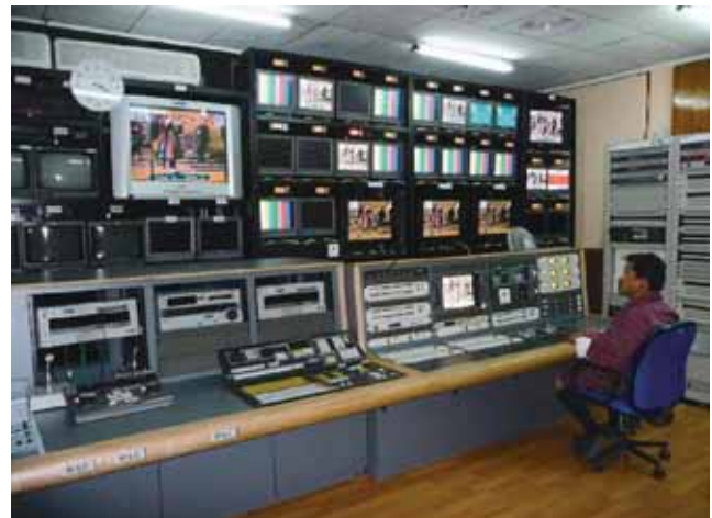
Master Control Room
