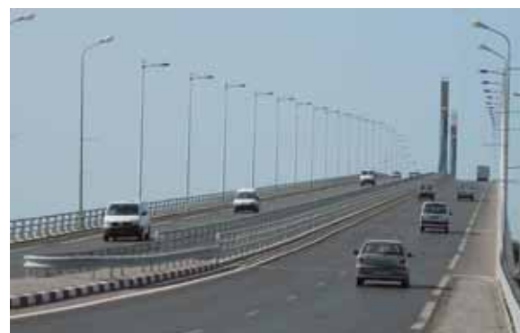
South Approach Bridge
