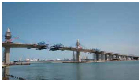
Main and South Approach Bridges under construction
