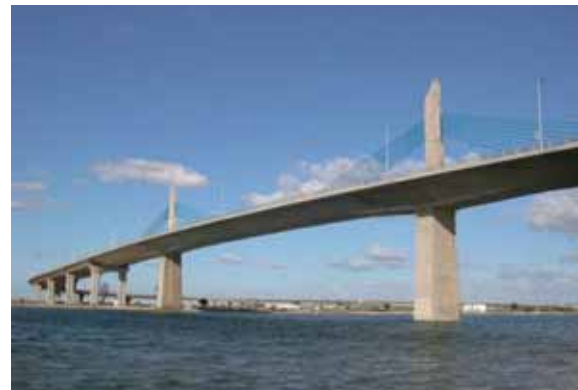
Main Bridge, North Interchange and Ramp Ways
