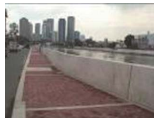
Construction of parapet wall.
