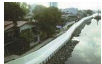
Installation of boulders as counterweight and protection against scouring.
