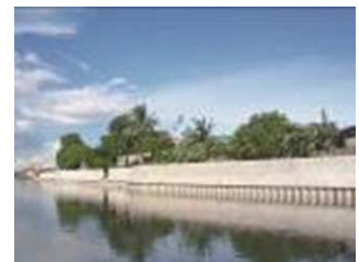
Installation of steel sheet piles.
