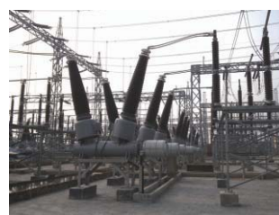
230kV AIS switchgear at Siddhirganj
