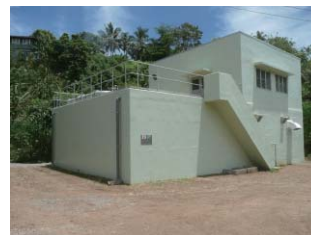
Water Transmission Pump Station
