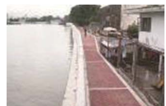
Clearing of the 3-meter easement of the River.
