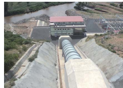
Powerhouse, Penstock and Switchyard
