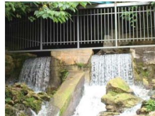
Main Watersource in Project Site
