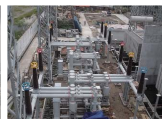
230kV GIS Switchgear at Maniknagar
