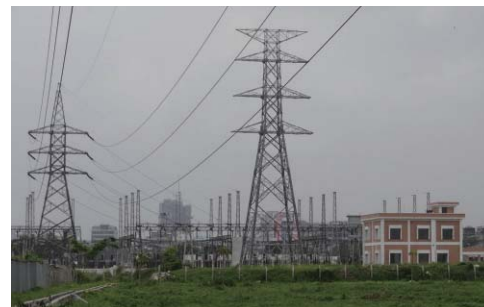
Maniknagar 230kV GIS substation
