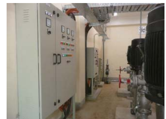
Transmission Pump Facility
