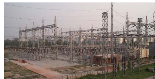
Siddhirganj 230kV AIS substation
