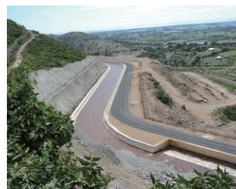
Additional Outlet Channel from Sondu-Miriu Power Plant (504 m)
