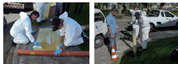
Demonstration of non-dig Pipe Rehabilitation Method
