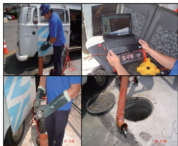
Field Investigation by Insert-Type TV Camera
