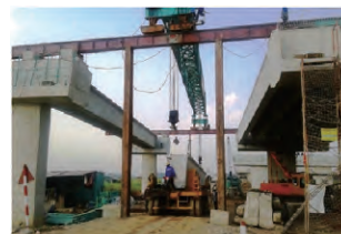
PC Super-T Girder Launching
