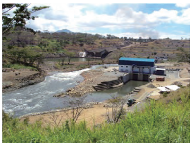
YTOD power station & tailrace channel
