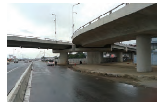
Ramp A and B
