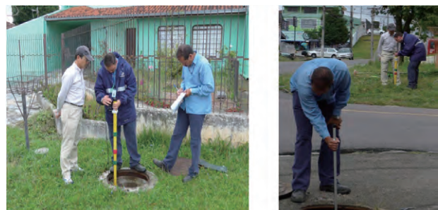
Field Investigation by Simple TV camera
