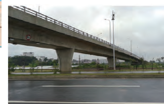
Flyover of Nam Hong
