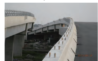
Flyover above Railway
