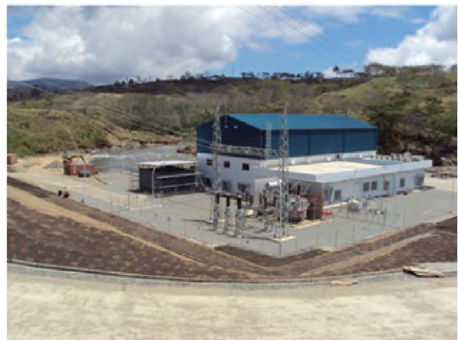
Outdoor switchyard & transformer
