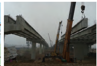
I-Girder Erection at Ca Lo Bridge
