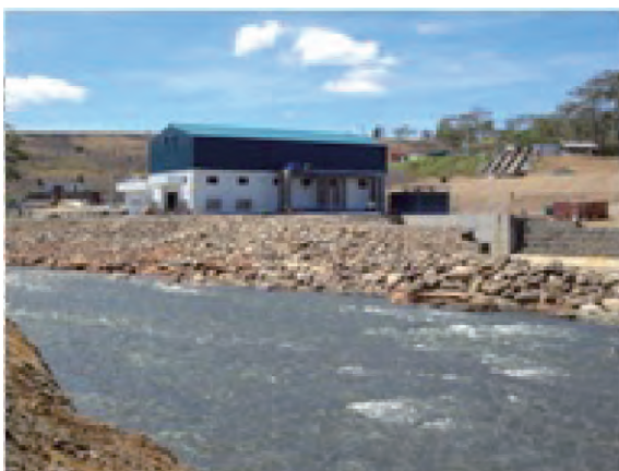
Bolder riprap against flooding
