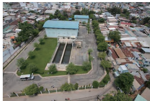
Intermediate Wastewater Pumping Station
