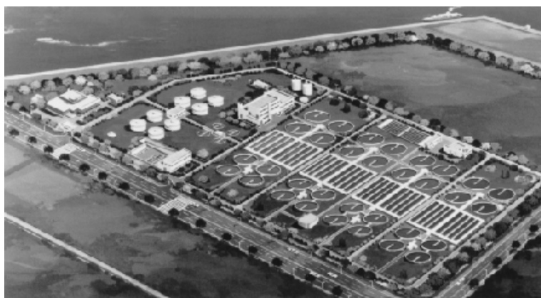
Kajoa Sewage Treatment Plant, Incheon City, Korea
