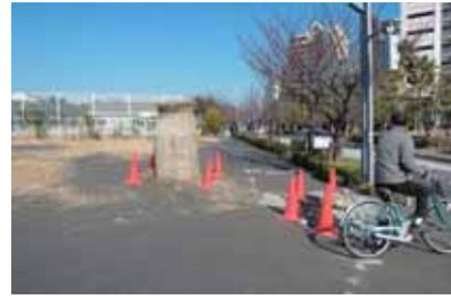
Uplifted manhole by liquefaction
