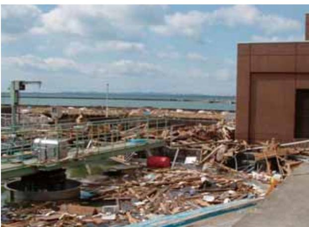
Sewage treatment facility blocked by a heap of rubble
