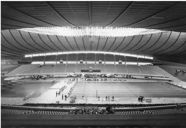
Picture 3 Interior of Stadium 1
