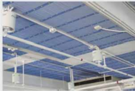
Radiant ceiling cooling system by capillary tubes
