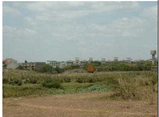
Expansion of urban area beside main road (A-109)
