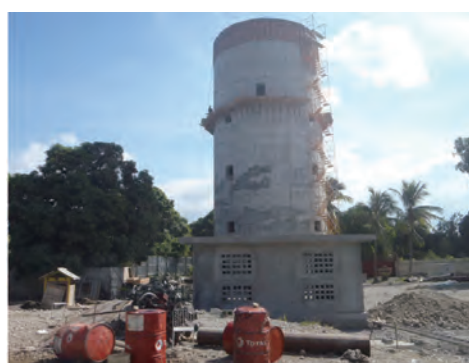
Photo Construction site of elevated tank
